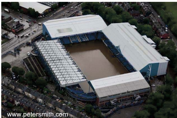
Flooding at Hillsborough stadium
