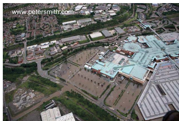
Meadowhall under siege from floodwaters
